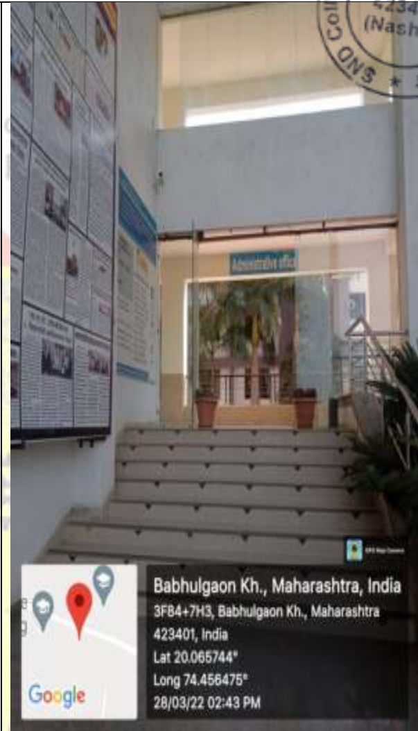
CCTV CAMERA AT ENTRANCE
